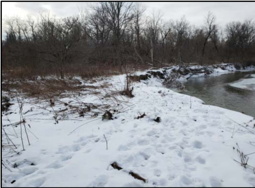
Figure 2. Eroded creek bank requiring bank stabilization work, facing upstream.
