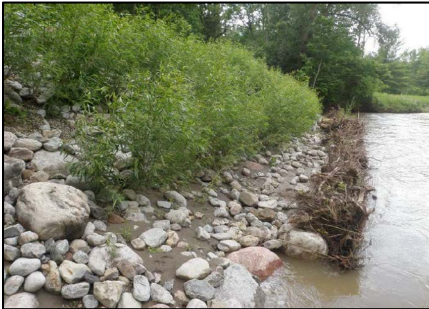
Figure 5 – Bank Stabilization
