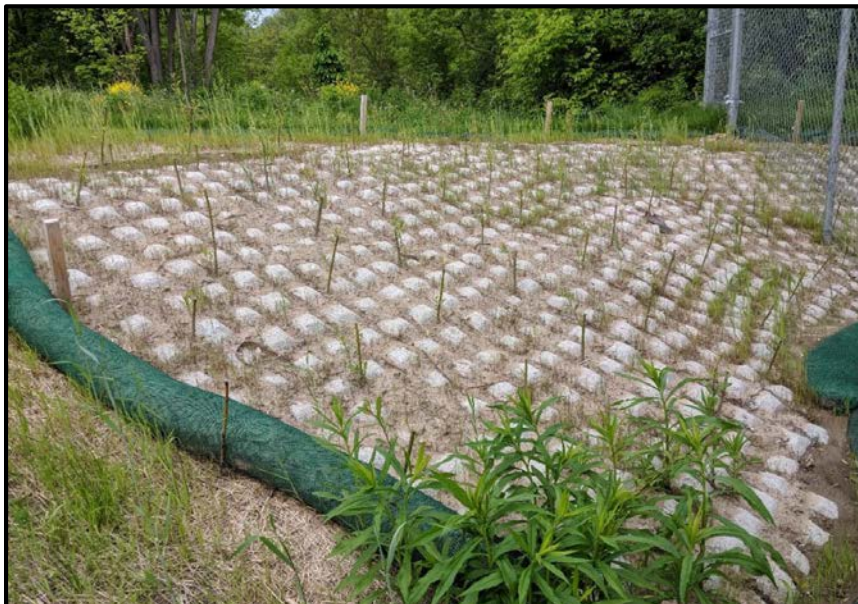
Figure 8 – Erosion control stabilization treatment - Flexamat
