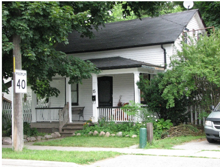
View from the southwest.
