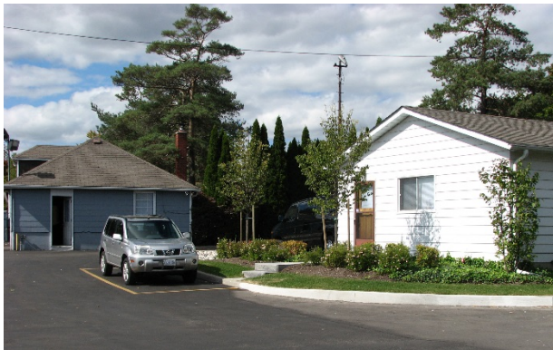
Rear outbuildings. The one on the right is recent. The one on the left may have been a stable/garage for the old dairy.
