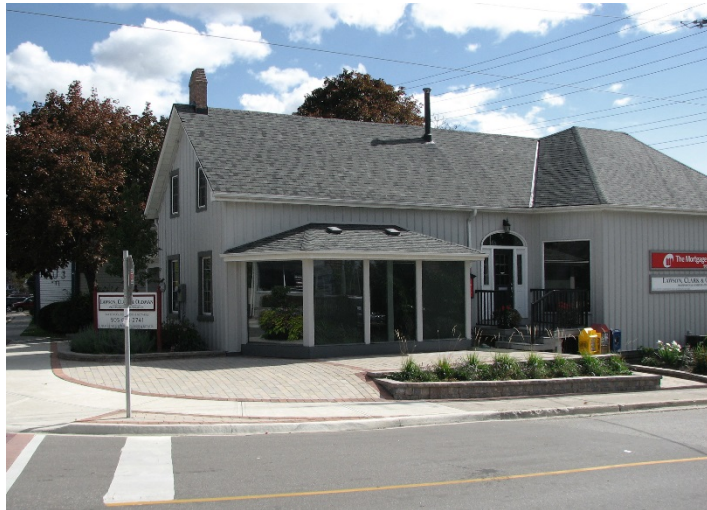
View from the west.
