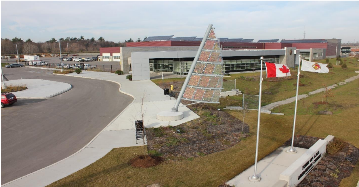
Figure 3: The Photovoltaic system (100kW) installed on the roof of Operations Centre.
